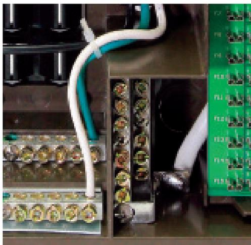
Built-in terminal bars for the negative DC wiring eliminate the time and cost of installing a separate negative DC bar.
